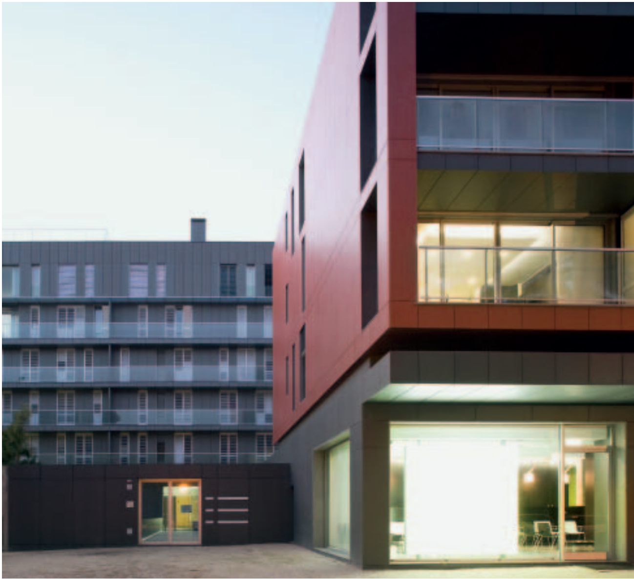
The two sections of the building are distinguished by red and pale grey, held together by the base floor clad in opal black. The upper end of the building, clad in titanium zinc, creates an additional material and colour nuance.
